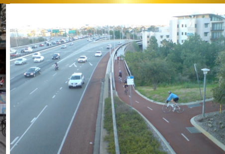
Painted Bicycle Lane on Major Urban Road
